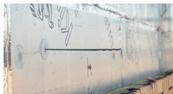
Dualfix Durable spouwanker positioneren
